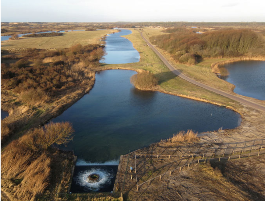
Fig. 12 Infiltration point of surface water from the lake IJsselmeer into the infiltration channels in coastal dunes area of Castricum. Photograph: T. Kisjes
