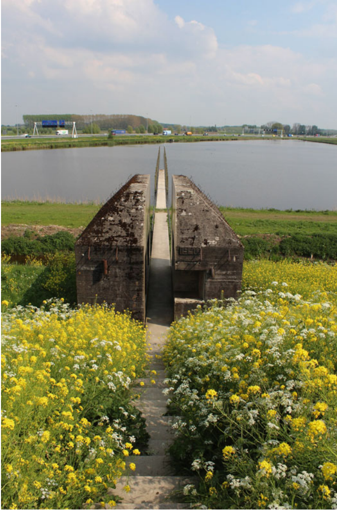
Fig. 6 Cut-through bunker 599 as part of the water storage and preservation of a bunker landscape. Courtesy Verschuure-Stuip 2014; released under a Creative Commons Attribution-NonCommercial-NoDerivatives 4.0 International License
