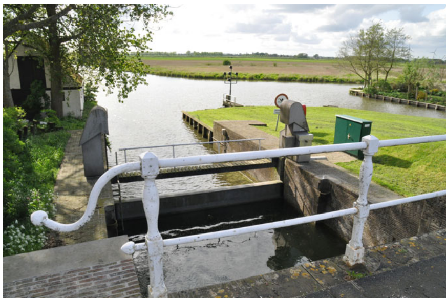
Fig. 17 Schardam, sluice (1592, Photograph: De Boer); released under a Creative Commons Attribution-NonCommercial-NoDerivatives 4.0 International License
