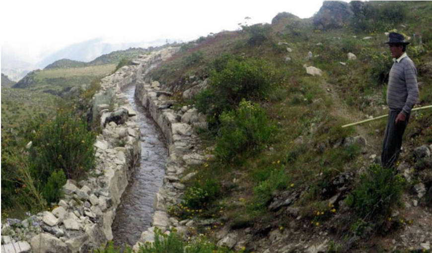
Fig. 5 Detail view of ancient mamanteo canal, part of a network restoration project being undertaken by SUNASS in Peru. Image courtesy of Leah Bremer/The Natural Capital Project; released under a Creative Commons Attribution-NonCommercial-NoDerivatives 4.0 International License
