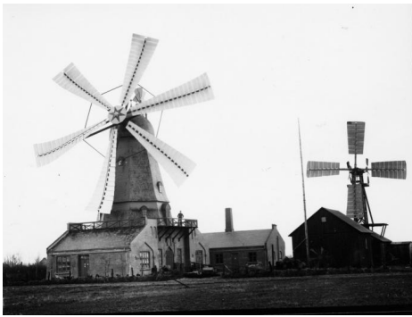
Figure 1.1: la Cour's experimental turbines at Askov, Denmark, as they stood in 1897. Source: Vejen Lokalhitoriske Arkiv.
