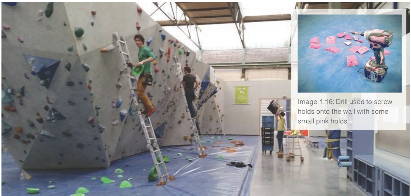
Image 1.17: Route builders at work using ladders and drills to screw the holds onto the wall. Routes are created during the screwing of the holds. Photo taken at Boulder centrum Delfts Bleau in Delft.
