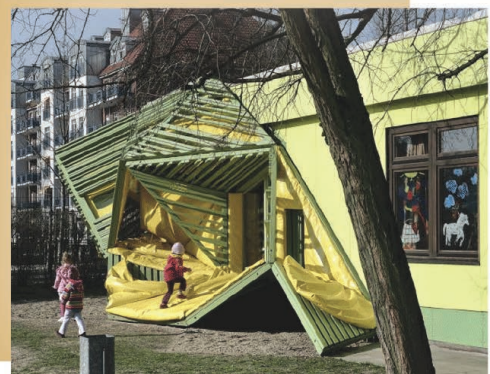
Outdoor playground with climbing rack integrated in the building.
