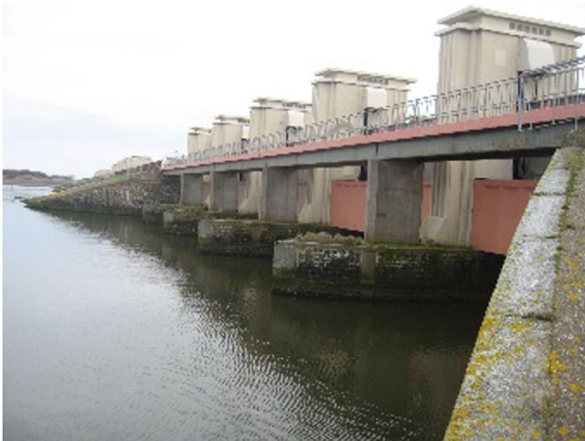
Figure 16. Discharge sluice in the closure dam (built 1932; source: beeldbank RWS).
