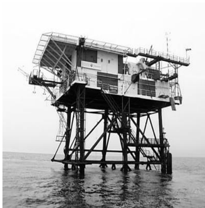
Figure A10-1 The Noordwijk measuring station
