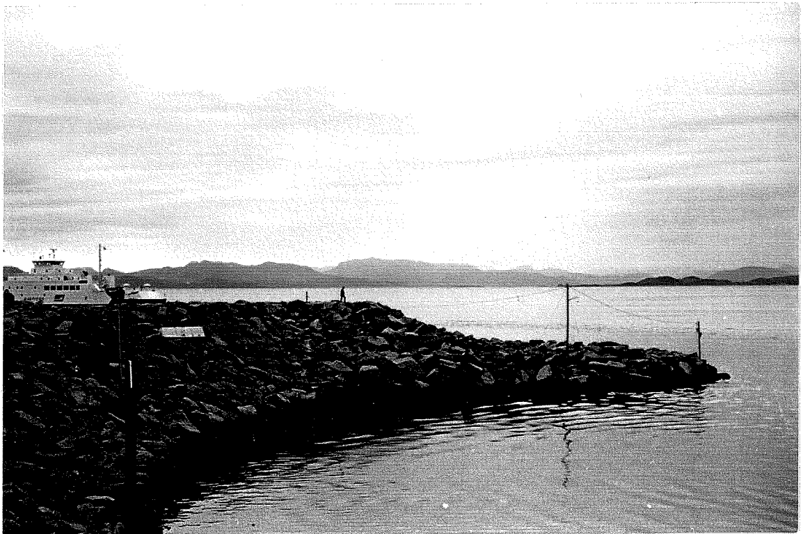
Figure 7 Photo of the Rennesøy breakwater head.
