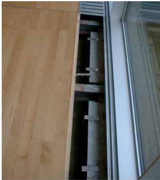
Figure 33: Grilles in the floor for the air inlet and the regulation of the airflow. (Hendriksen, Brohus, Frier, & Heiselberg, 2002)
