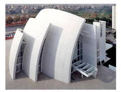
Fig. 1 Jubilee Church, Rome (architect: Richard Meier), double-curved elements in precast concrete
