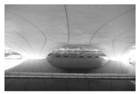
Fig. 2 Spencer Dock Bridge, Dublin (architect: Future Systems), cast in site concrete using double-curved formwork
