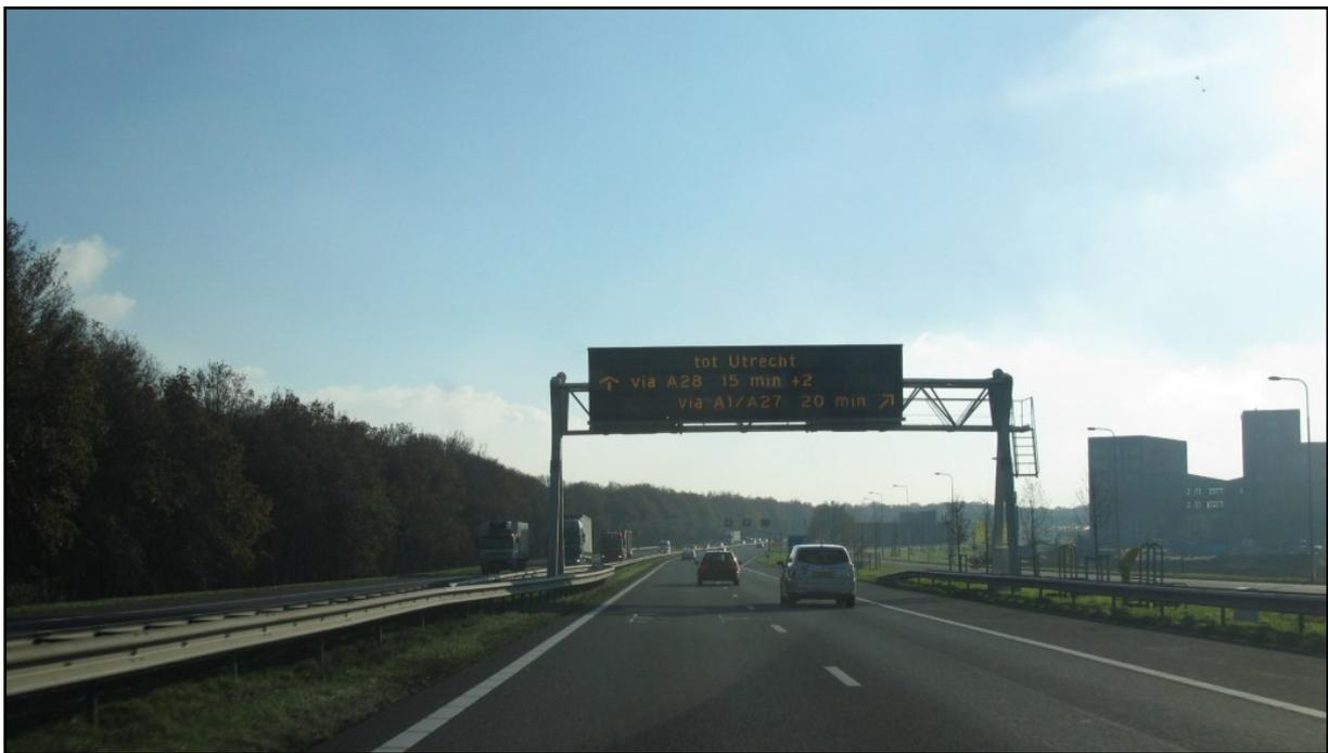
**Figure 2.6 Example of a VMS in operation: it shows the travel time + delays via two alternative routes to the city of Utrecht (Source: [Chriszwolle, 2010](#))**
