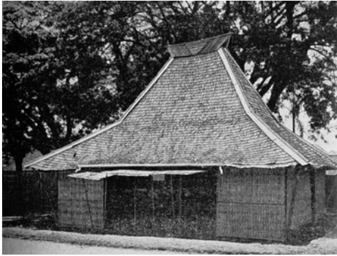
Traditional dwelling according to a design created by the engineer H. Maclaine Pont in order to illustrate his lecture 'How can the endeavour to improve the housing situation in Java be turned into a national movement?' (1925)
