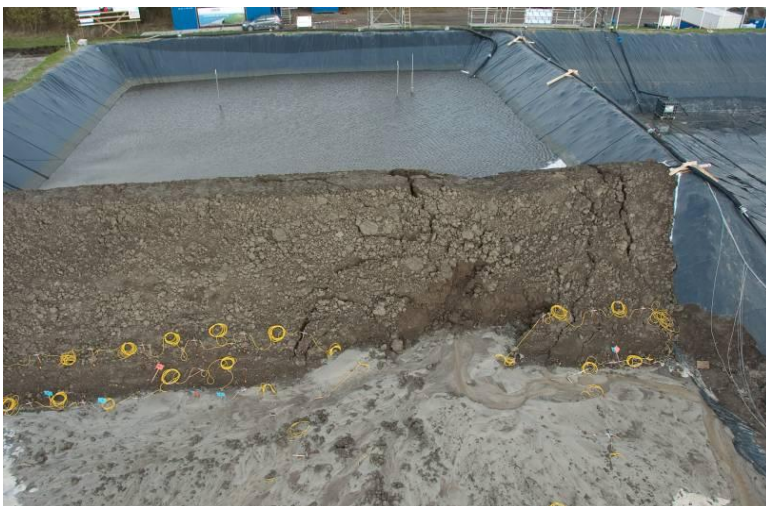
Figure 9: Failed dike in full-scale field experiments. The dike is 3 m high and 15 m wide. Water level was increased until 2.5 m.
