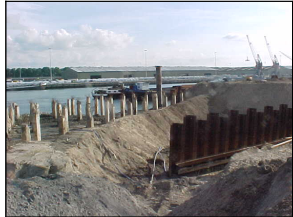
Fig. 4 Anchor wall and reused foundation piles
