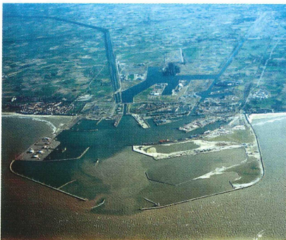
Fig. 2: Continuous dredging is required maintaining navigable depth in Zeebrugge, Belgium.
