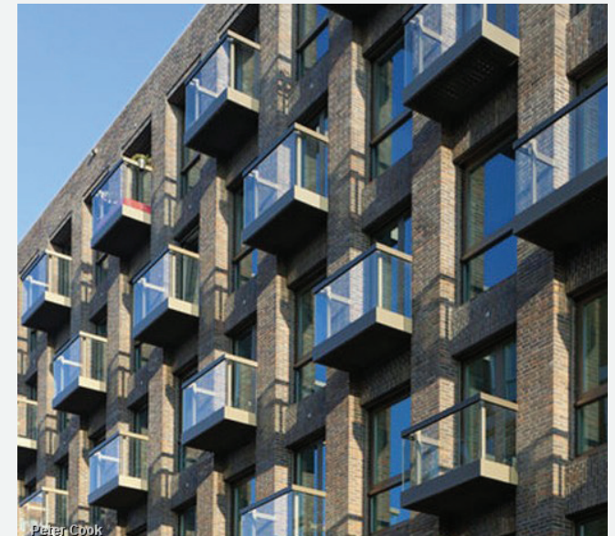
Image 3.10.3: New Façade of the former Wilhelmina Gasthuis in Amsterdam (INBO, s.d.).
