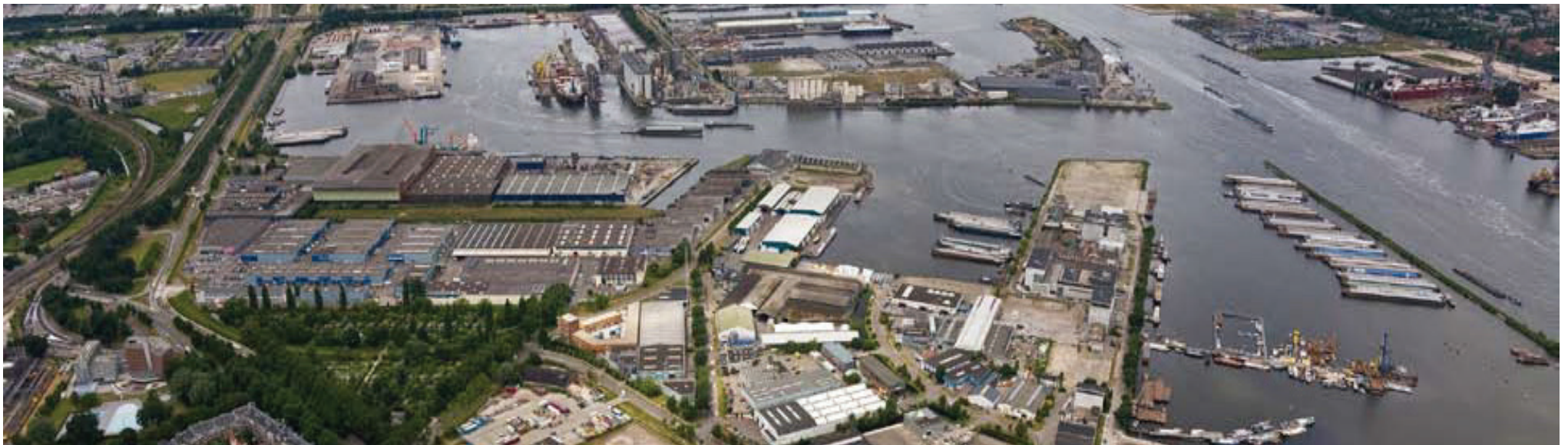
Image 1.2.7: Aerial picture of the project site in Amsterdam showing the Minerva City-harbour and the Coen- and Vlothaven (DRO and Haven Amsterdam, 2009: 34).
