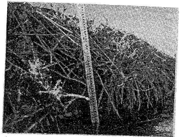
Photo 1: A bank with a protruding upper soil layer
