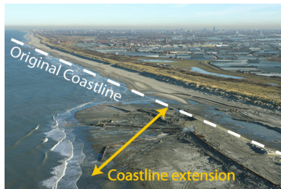
Figure 4. Aerial picture of dredging works showing the significant coastline extension.
