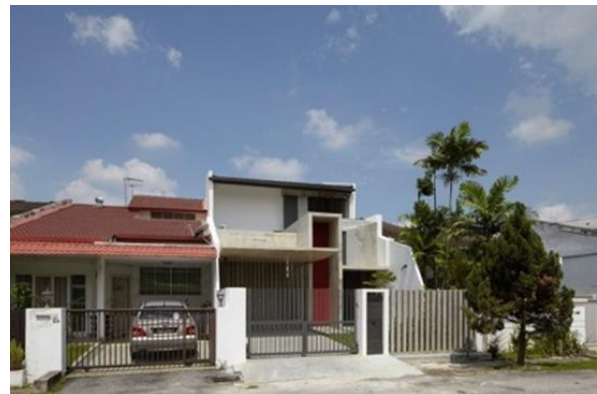
Fig. 5. The renovation has involved a frontal extension and changing of the roof structure to accommodate bigger master bedroom
