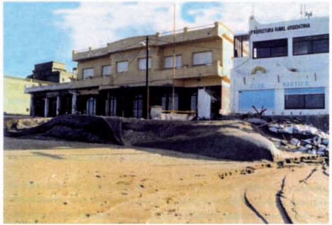
DISASTROUS SITUATION MUNICIPALIDAD DE LA COSTA: 1 x MAR DE AJO & 4 x MAR DEL TUYU THE PRIMARY RANGE OF DUNES WAS LEVELLED FOR HOTELS & SEASIDE PAVILIONS. WRONG JUDGEMENT !! THE CONSTRUCTION OF SOLID SEAWALLS DIDN'T HELP, THEY ONLY AGGRAVATED THE PROBLEM.
