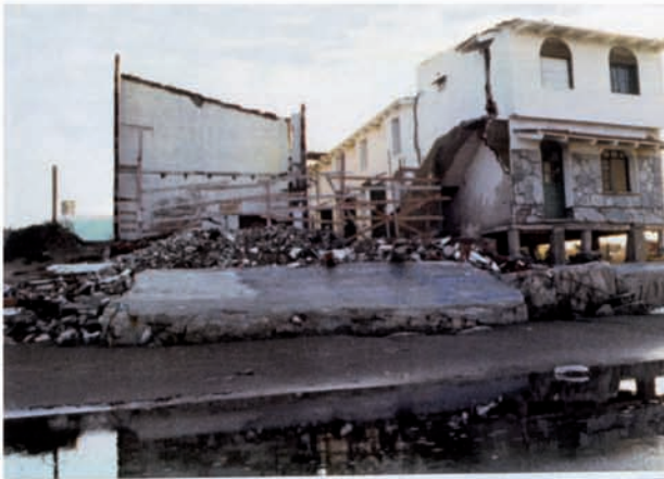
DISASTROUS SITUATION MUNICIPALIDAD DE LA COSTA: 1 x MAR DE AJO & 4 x MAR DEL TUYU THE PRIMARY RANGE OF DUNES WAS LEVELLED FOR HOTELS & SEASIDE PAVILIONS. WRONG JUDGEMENT !! THE CONSTRUCTION OF SOLID SEAWALLS DIDN'T HELP, THEY ONLY AGGRAVATED THE PROBLEM.
