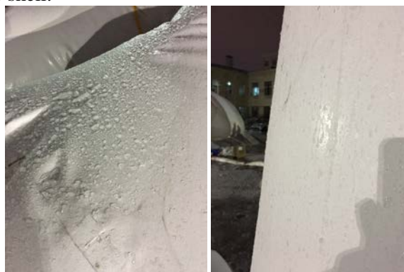
Figure 17: Attached ice on the inflatable mould
