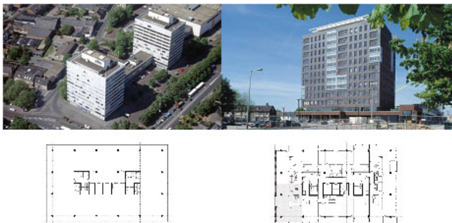
Figure 2 The Twentec building, another of the building transformations we studied ex-post. Left the building before conversion, to the right the building after conversion. The project was part of a larger restructuring of the city centre of Enschede, and one tower was demolished to allow for a large underground parking garage to be built. The other tower was transformed into housing.
