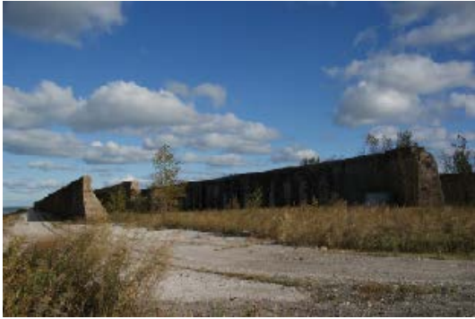
Condition of Ore Walls
